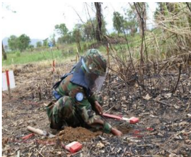
Demining worker Mrs. Mot Huot carefully uses a prodder to probe an area suspected to contain a landmine in a Clearing for Results project minefield in Pailin province. (Photo: CMAA/Art Veasna)
